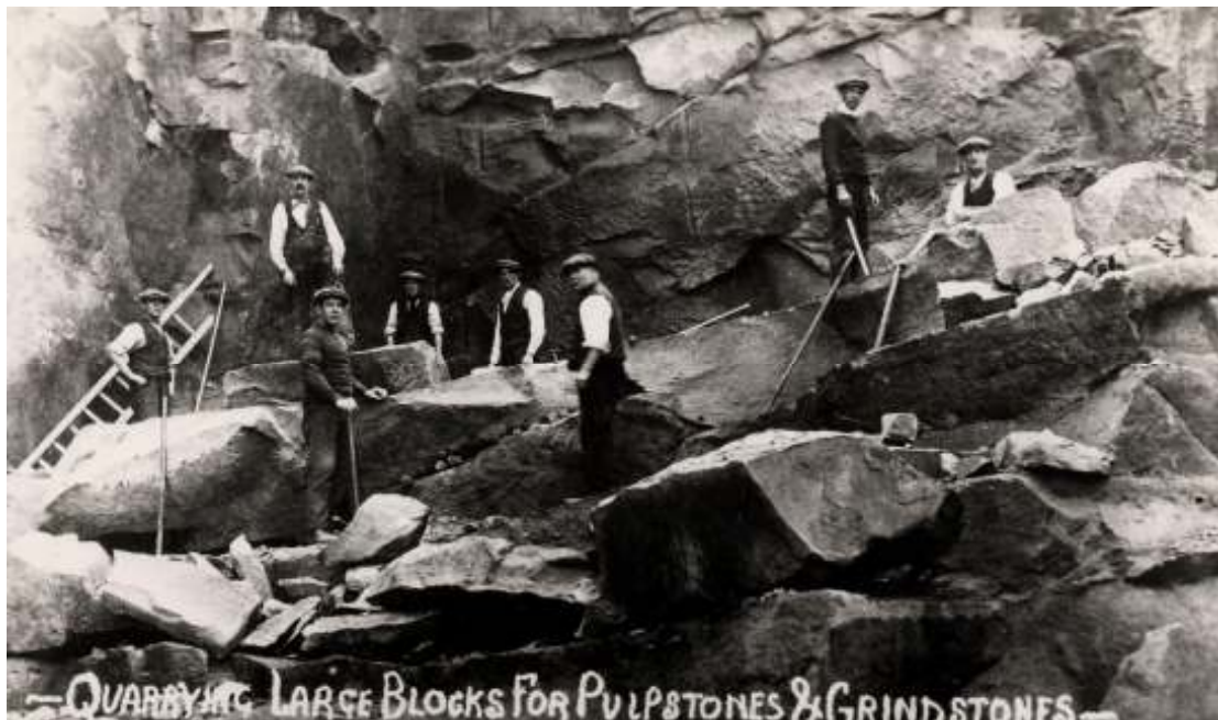
Quarrying blocks for pulpstones and grindstones, Windy Nook Quarry
